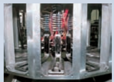
Interior of center column
